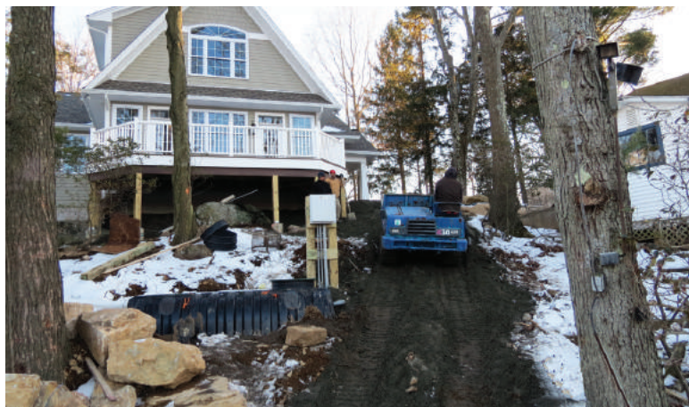
Avery Jinks of Septic Experts eases the IHI 1.3-cubic-yard IC30 crawler carrier up the steep slope past the septic tank and control panel to deliver another load of bank run.
